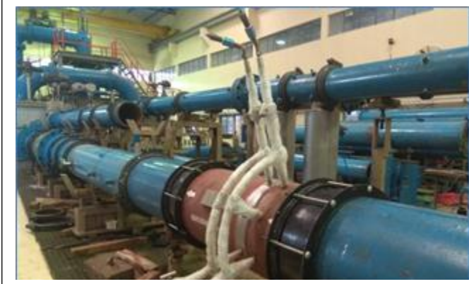
20" NB cone flowmeter under Calibration
