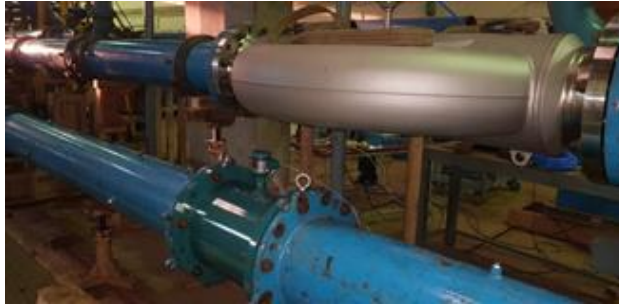
Calibration of 12" magnetic flow meter at WFL
