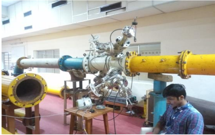
Calibration of 10" NB Ultrasonic flow meter at Air Flow Laboratory
