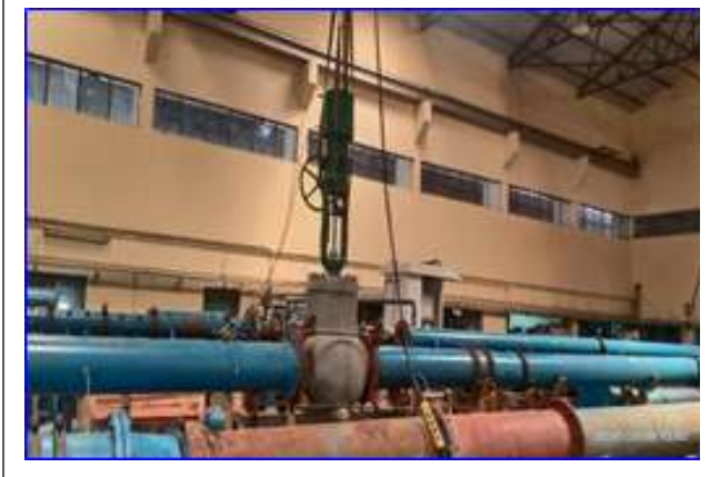
Testing of 6" angle valve at WFL
