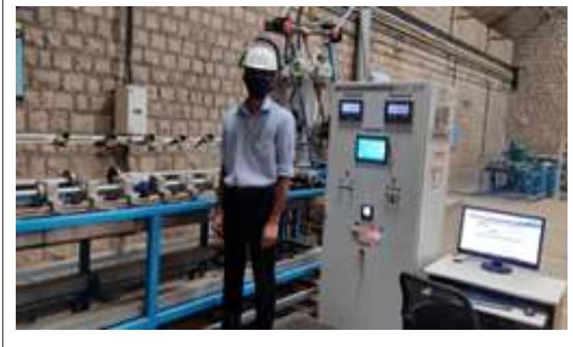
AMR (Automated Meter Reading) testing of DN 15 water meter
