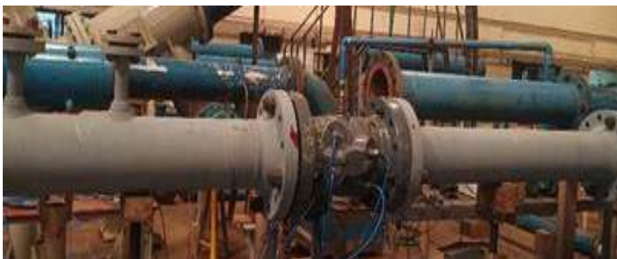
Calibration of inline ultrasonic flow meters of size 12" at WFL
