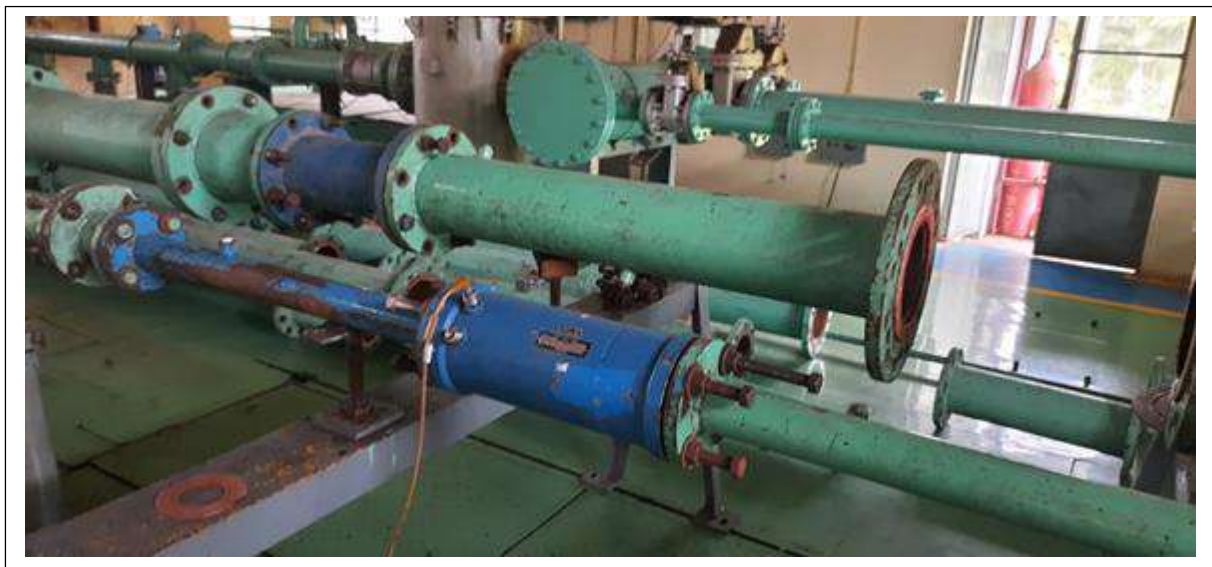
Calibration of PD meter of size 3" at OFL
