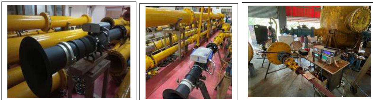
Calibration of flow meters at Air Flow Laboratory
