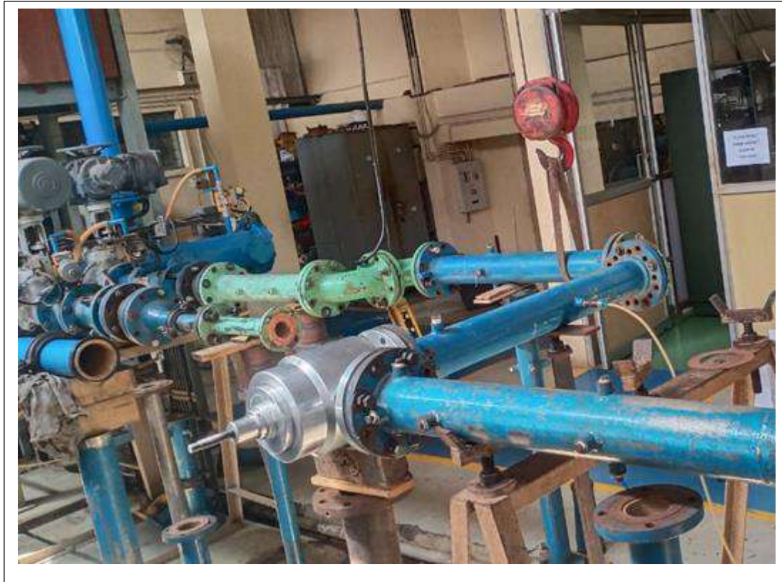
Testing of 4" angle valve at WFL
