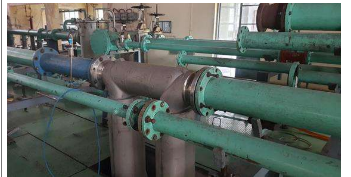
Calibration of Mass flow meter of size 6" at OFL
