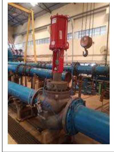
Testing of valve of size 16” at WFL
