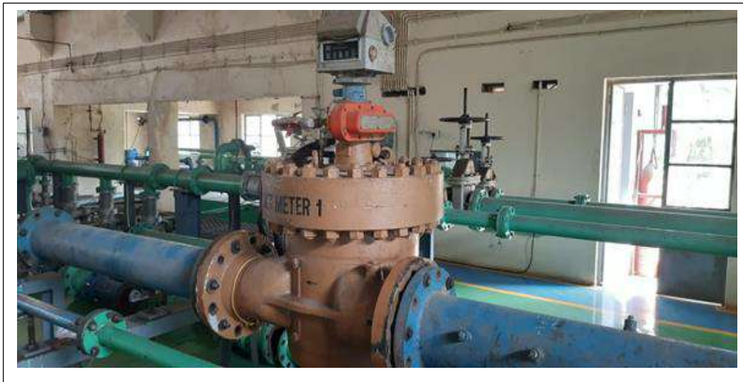
PD flow meter Calibration at OFL
