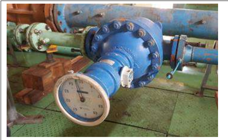
Calibration of PD flow meter at Oil Flow Laboratory
